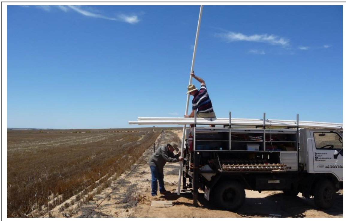
Figure 4 Installation of piezometer well tubing at Site MDS-P05.
