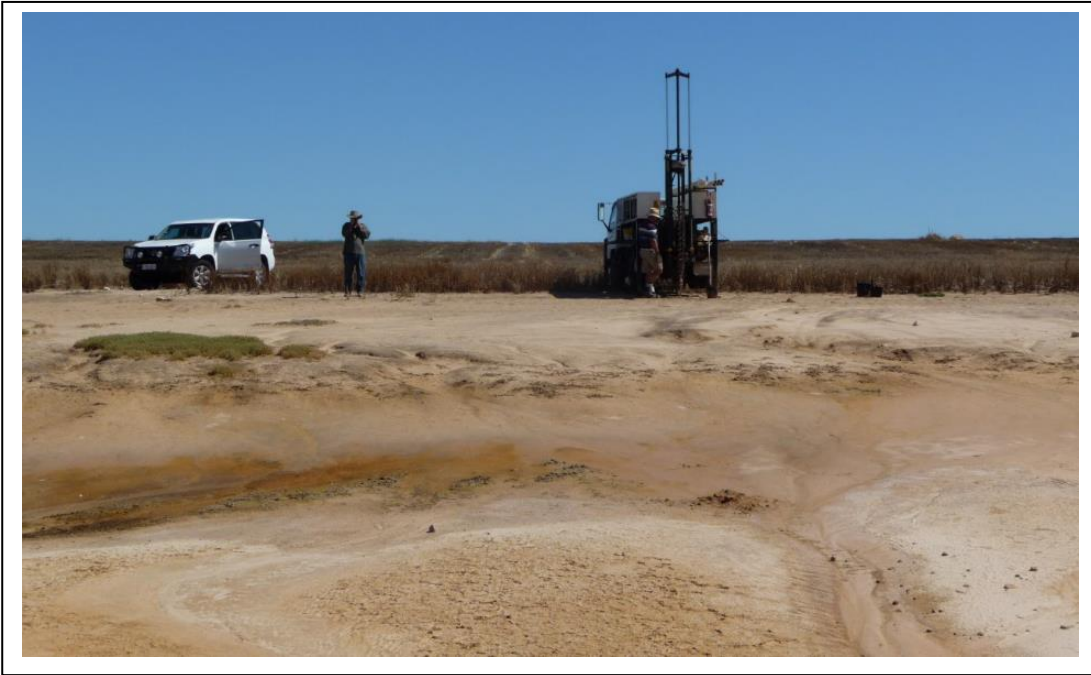
Figure 8 Drilling at Site MDS-P07 – looking upslope.
