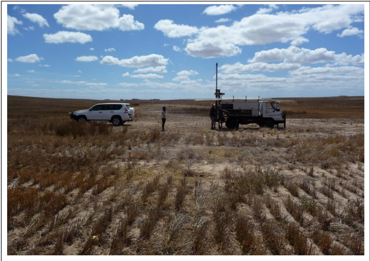
Figure 9 Drilling at Site MDS-P09.
