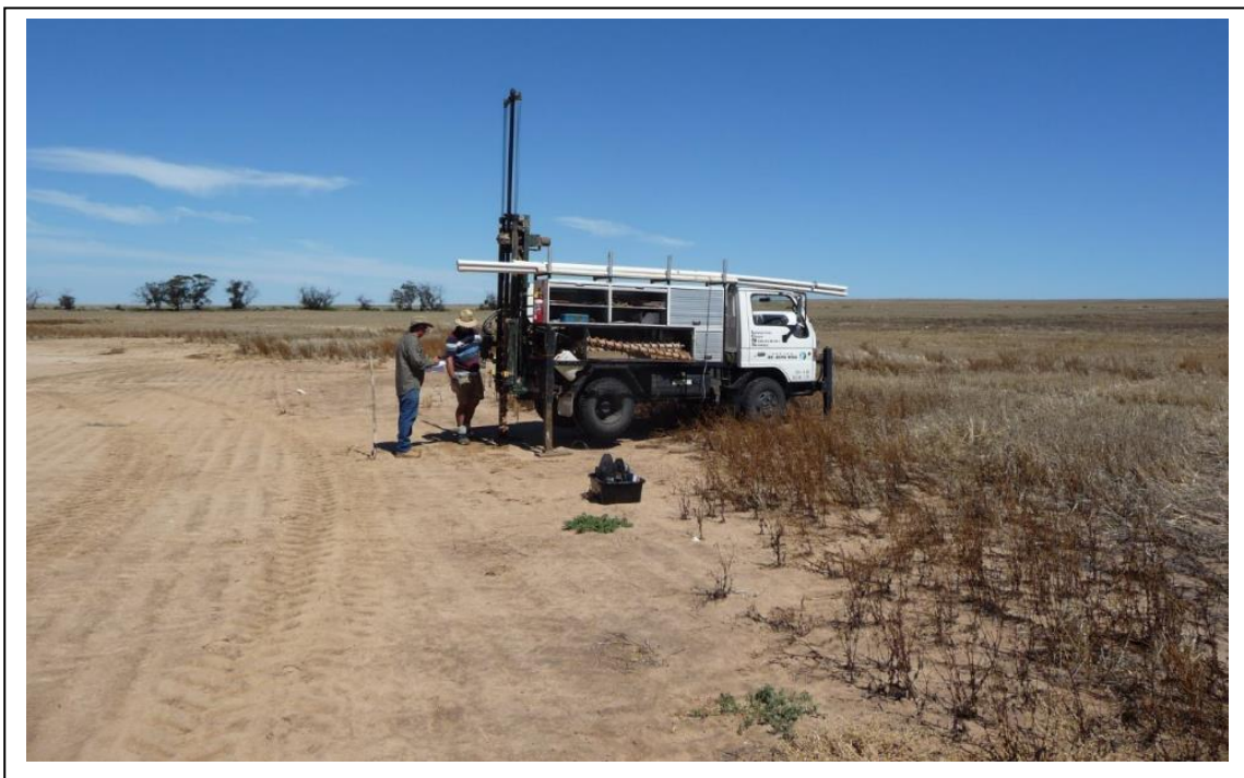
Figure 6 Drilling at Site MDS-P07.
